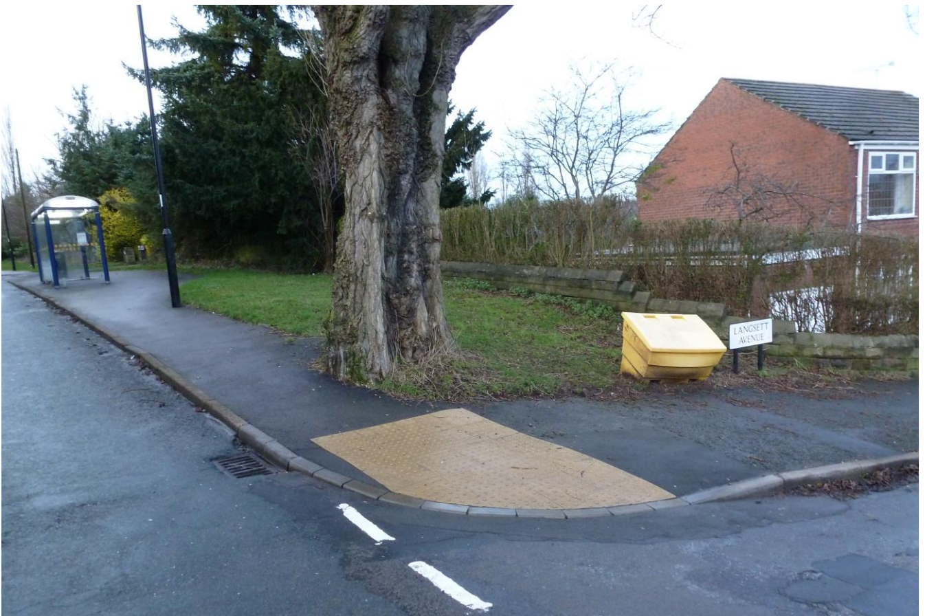
24 th January, 2016. The Wadsley poplar; the toxic “grit bin” (rock salt) and the “ significant ” footway damage. The knobby, beige surface at the junction was added between May & December, 2015.
